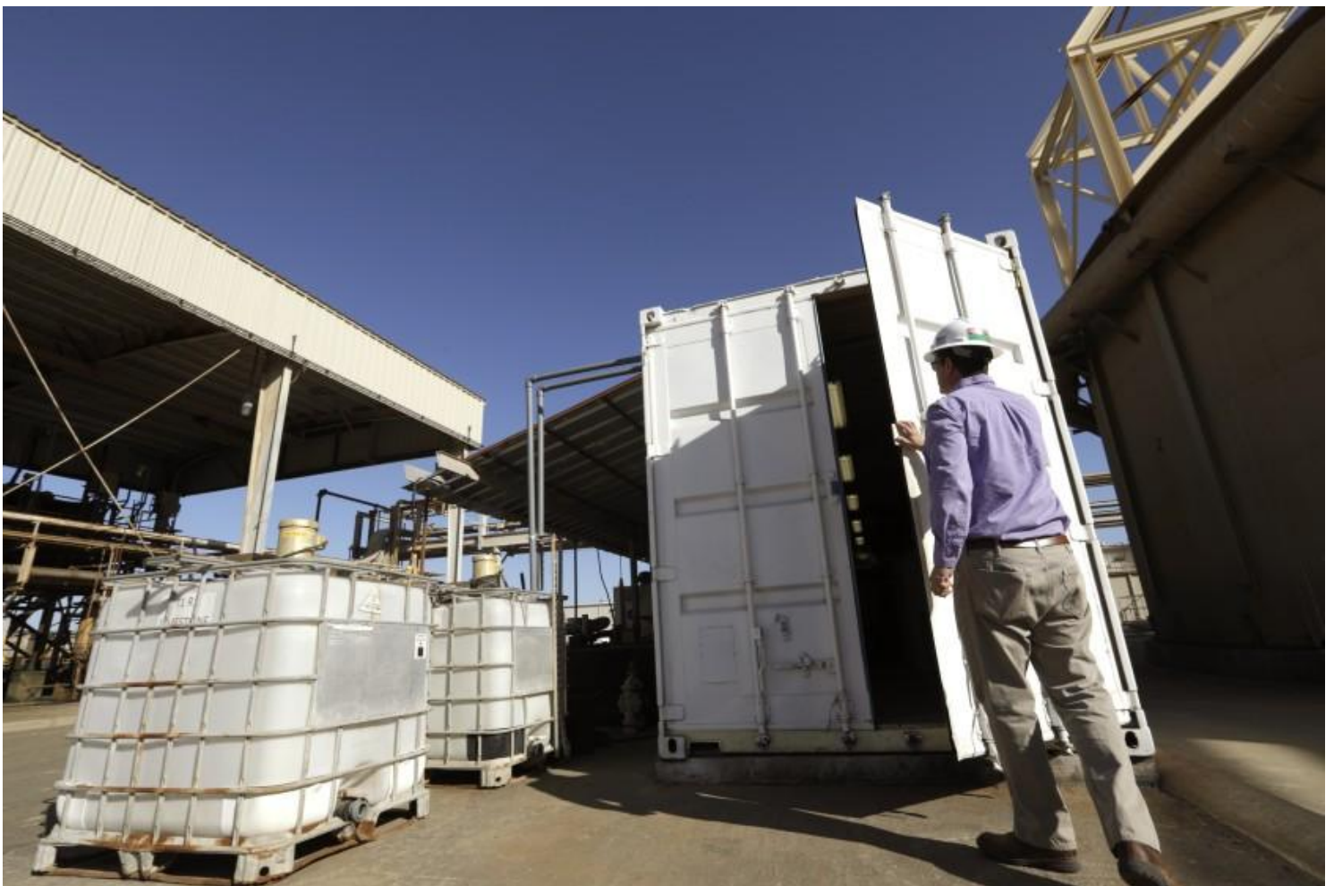
EnergySource Chief Operating Officer Derek Benson opens a shipping container at the company’s John L. Featherstone geothermal plant near the Salton Sea. Inside the container is equipment for the company’s lithium extraction process. (Carolyn Cole / Los Angeles Times)
