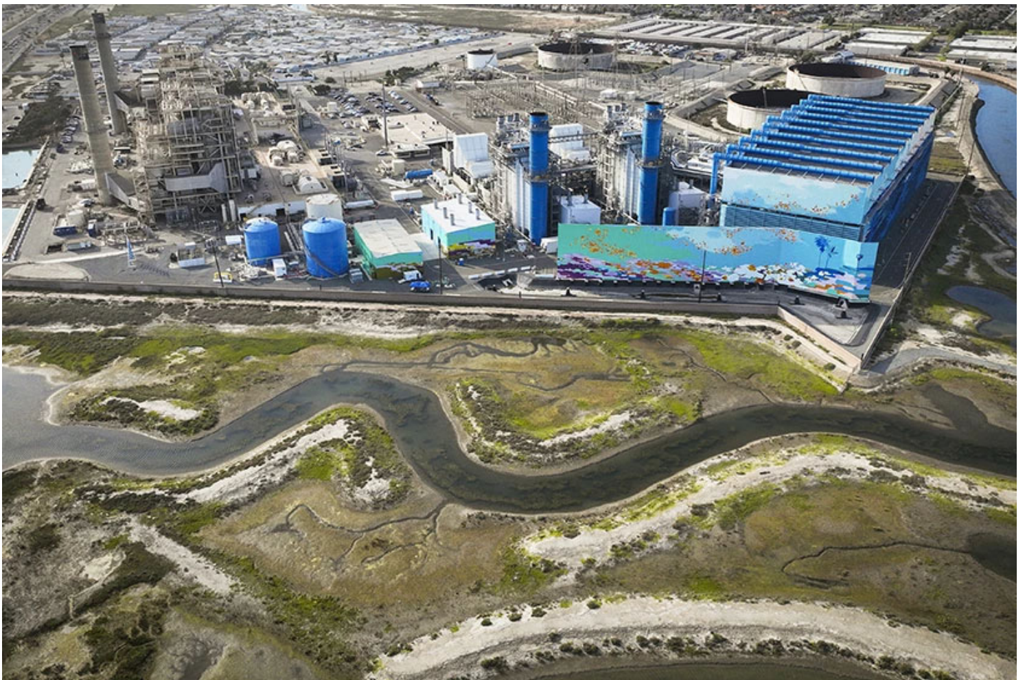
The Huntington Beach Generating Station includes a natural gas generator that began operation in 2020. (Allen J. Schaben / Los Angeles Times)
